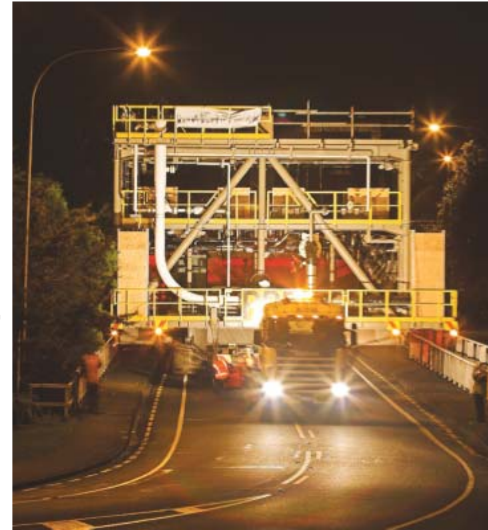
The transporter inches the topside module across the Te Henui Bridge.
